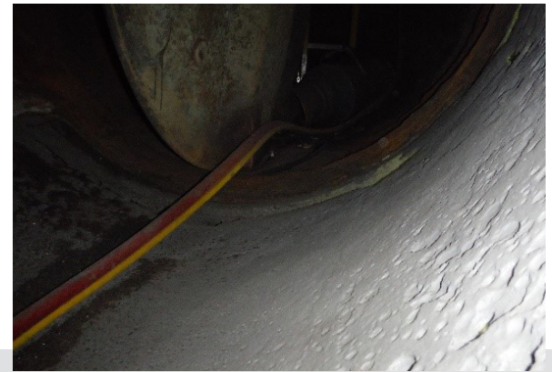
Figure 1 Deep Pitting in Host Pipe
