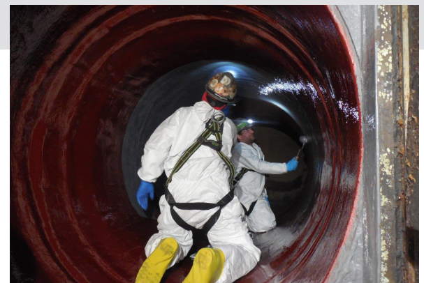
Figure 3 Application of HP-300 Epoxy
