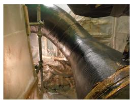
After: The carbon fiber pipe repair system was installed on-time and on-budget during a busy plant outage. The system is engineered to withstand more than double the design pressure of the original circulating water line. This composite pipe repair will provide a 50-year, maintenance-free service life, even in aggressive saltwater immersion conditions.
