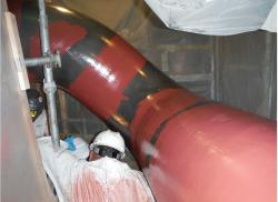
During: Advanced FRP Systems designed a structurally independent carbon fiber composite pipe with a flange-to-flange wrap design, to completely rebuild this section of piping. The external application of the composite allowed the repair to be done without draining the circulating water line, minimizing the required downtime for the repair.
