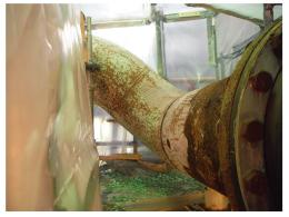
Before: A New York power generation facility was experiencing systemic corrosion in their circulating water lines. A section of 30-inch diameter, carbon steel pipe was experiencing internal and external corrosion and required immediate attention. Instead of pipe replacement, a composite pipe repair was chosen to provide a 50-year life extension.
