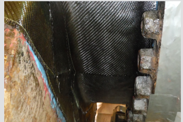
Figure 2 Carbon Fiber Wrapping
