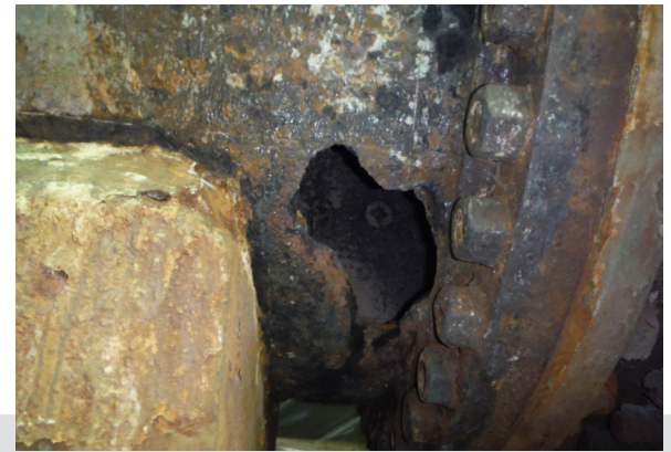
Figure 1 Pipe Before Repair
