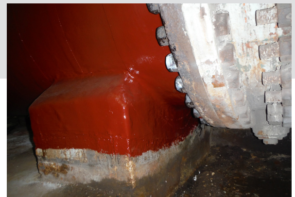
Figure 3 Application of HP-300 After Repair
