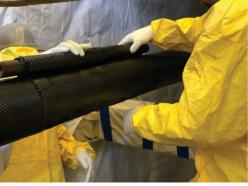
During: After excavating and identifying adhesion zones, our carbon fiber composite reinforcement system was applied to both the feeder and return lines while still online. The adhesion zone concept eliminated 90% of the surface preparation while encapsulating 100% of the pipes with a structurally independent composite.
