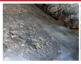
Before: A New York-based utility found systemic corrosion in their underground HPFF transmission system. The corrosion rate was significantly accelerated in certain areas due to stray current. Though externally welded sleeves were applied during previous repairs, new dielectric fluid leaks began to occur after only 3-5 years.
