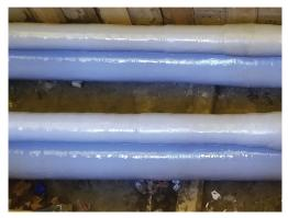
After: The system will provide a 50-year, maintenance-free service life verified to withstand more than 1,000 psi of internal pressure, even with a through-wall failure in the host pipe. The high thermal conductivity of the carbon fiber composite allows the system to stay well within the operating margin of safety for heat transfer.
