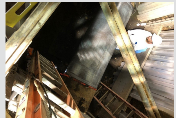
Figure 2 Application of Adhesive
