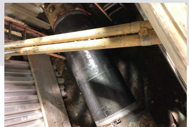
Figure 3 Final Carbon Fiber Repair
