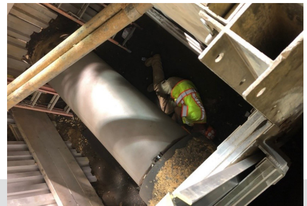
Figure 1 Pipe Surface After Grit Blasting
