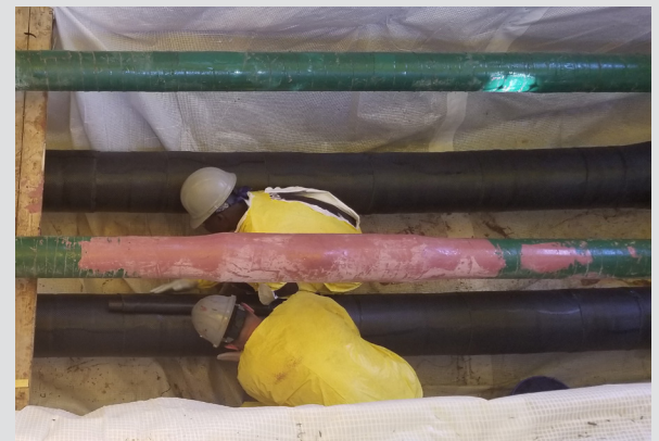
Figure 2 Installation of CF Composite
