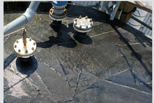
Figure 2 Carbon Fiber Installation on Tank Roof
