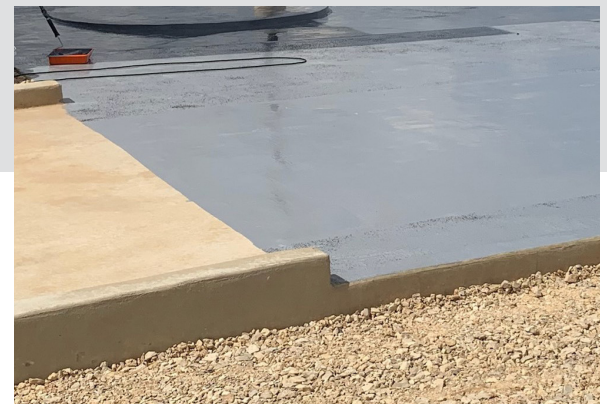
Figure 3 Close-up of Non-Slip Finish on Walkways
