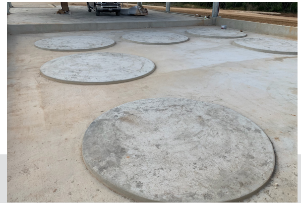
Figure 1 Concrete Containment Area Prior to Coating
