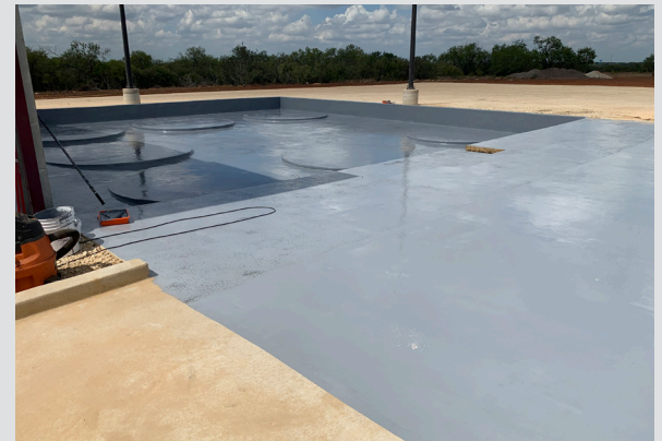
Figure 2 Fill Station After Final Coat of HP-400 Novo
