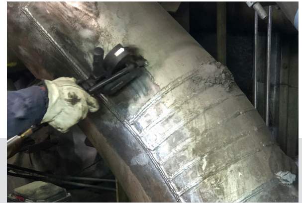
Figure 1 Bristle Blast Surface Preparation over Previously Repaired Elbow
