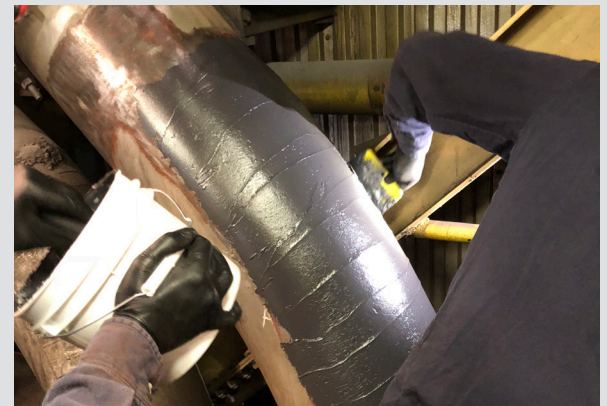
Figure 2 Application of Ceramic Repair Putty over Extrados of Elbow
