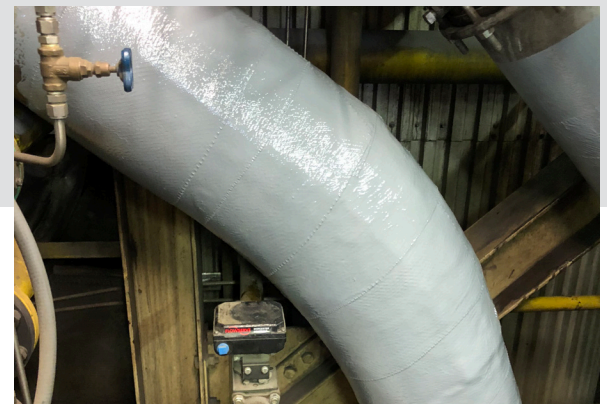
Figure 3 Coal Pipe Elbow After Installation of CF Composite and Topcoat
