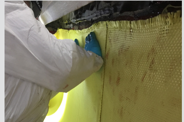
Figure 2 Installation of the Kevlar Reinforcement Fabric
