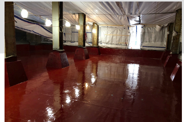
Figure 3 Final Basin After Application of the HP-300 Elastomer
