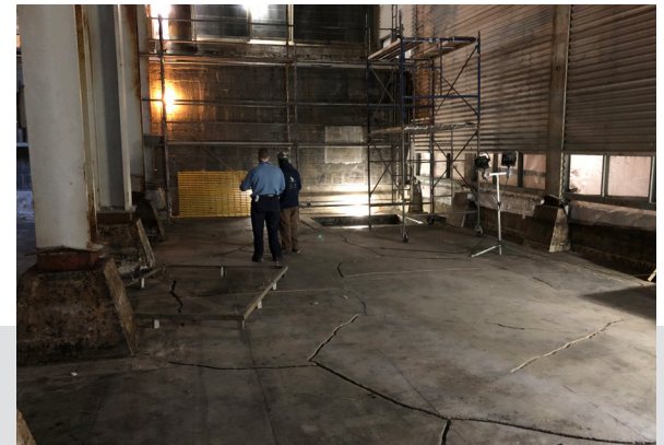
Figure 1 Cracks in the Concrete Basin Floor After Removal of the Tile Liner
