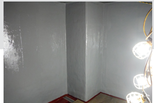
Figure 3 After Application of Second Coat of HP-400 Novo Topcoat
