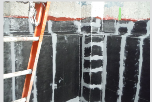
Figure 2 Carbon Fiber Reinforcement Applied over Edges and Corners
