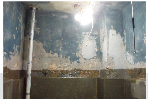
Figure 1 Tank After Application of FRP 200 Sealer to Bottom Half
