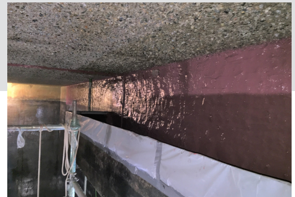
Figure 3 After Application of Two Inches of EM-110, High-Strength Epoxy Mortar
