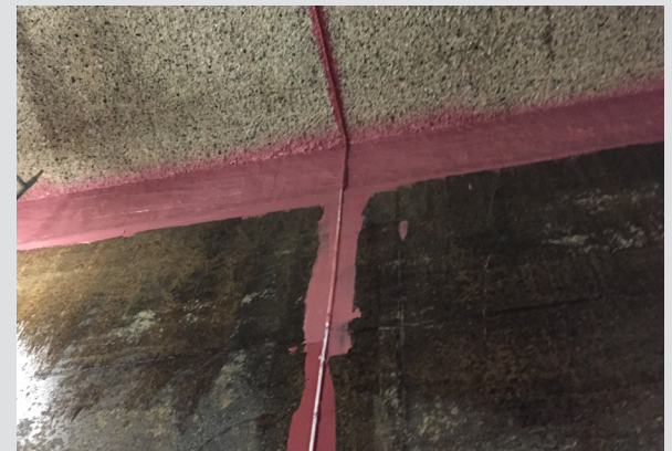
Figure 2 Temporary HDPE molds to rebuild Expansion Joint
