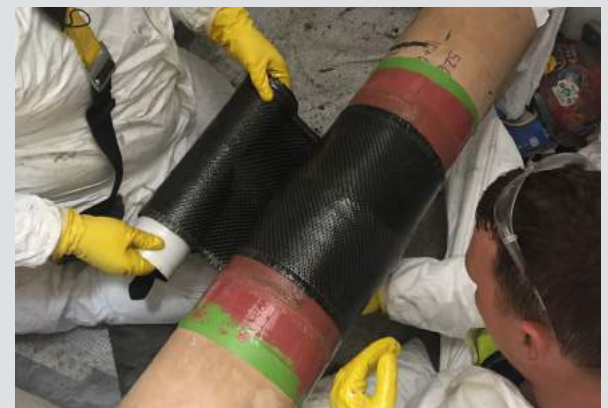
Figure 2 Application of Carbon Fiber Composite over the 8-inch Feeder Pipe
