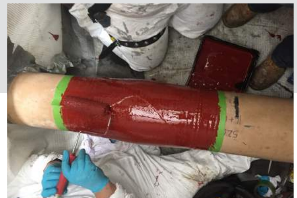
Figure 3 Application of HP-300 Topcoat System Prior to Holiday Testing
