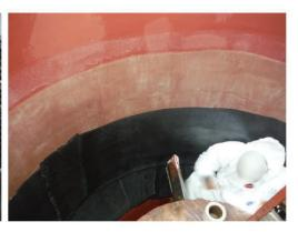
Full Tank Enhancement: A full tank reinforcement system was installed to repair severe degradation from microbially induced corrosion. Coupled with a ceramic-reinforced epoxy, the composite system was chosen to reinforce and protect the existing tank instead of replacing it.
