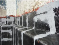
Tank Wall: A chemically-resistant carbon fiber composite installed on a concrete overflow tank containing 95% sulfuric acid. Inspections revealed many through-wall failures where previous coatings had failed. The composite was easily installed over the tank's unique geometry.
