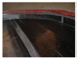
Tank Floor: A high-temp carbon fiber composite repair was performed on the floor of a condensate tank with through-wall failures. The complete system, including a permeation-resistant topcoat, was installed and fully cured in only 7 days during a short plant shut-down.
