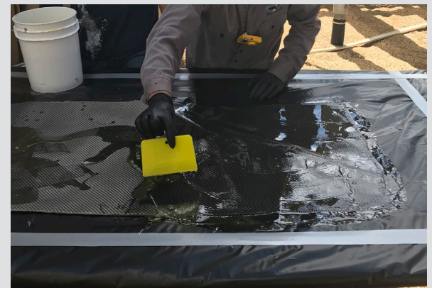
Figure 2 Saturation of the 25-inch width Carbon Fiber Fabric
