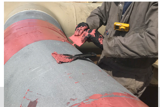
Figure 1 Smoothing of the Pipe and Weld Seams with FRP Repair Putty
