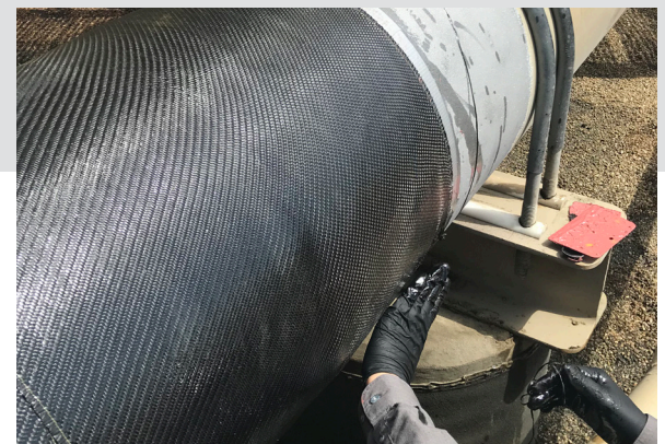
Figure 3 Application of Carbon Fiber Composite Reinforcement
