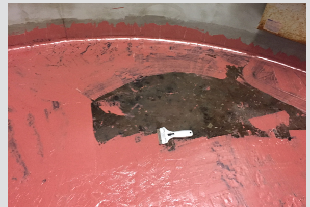
Figure 2 Pitting Repair with FRP Repair Putty Prior to Glass Reinforcement
