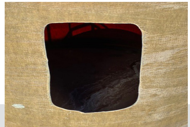
Figure 1 Tank with Large Cut-out for Access
