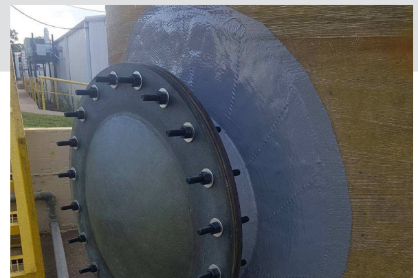
Figure 3 Final Repair After HP-300 Topcoat Application
