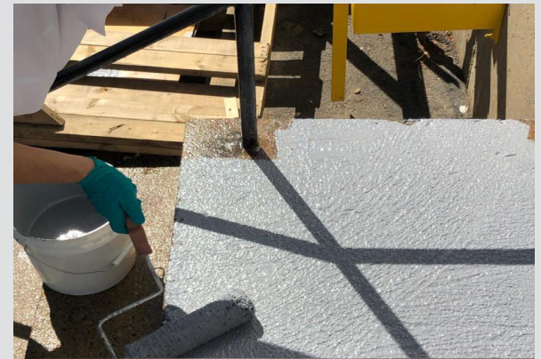
Figure 2 Application of HDF-250 AS Via Roller
