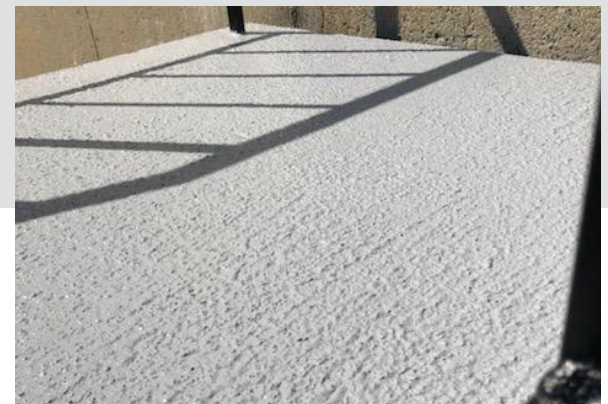
Figure 3 Staircase After Curing of HDF-250 AS
