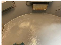
An underground pumping vault frequently filled with groundwater contaminated with road salts causing the previous coating to completely fail and allowed through-wall failures to develop. HP-300 Elastomer was installed to provide excellent resistance to intermittent water-immersion and physical abuse from maintenance activities.
