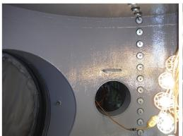
A condenser waterbox was experiencing extreme corrosion due to a failed coating system with the most significant corrosion on the hot side of the condenser. HP-300 GF was installed to provide long-term protection in operating temperatures up to 120°F and was compatible with the existing cathodic protection system.
