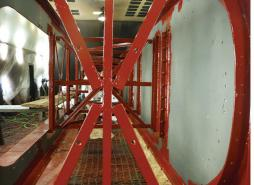
A traveling water screen at a power generation facility was experiencing rapid corrosion as a result of Microbially Influenced Corrosion. HP-300 Epoxy was applied successfully, pinhole-free, despite the complexity of the unit. HP-300 Epoxy reduces the accumulation of microbes on the surface and protects from chemical attack.
