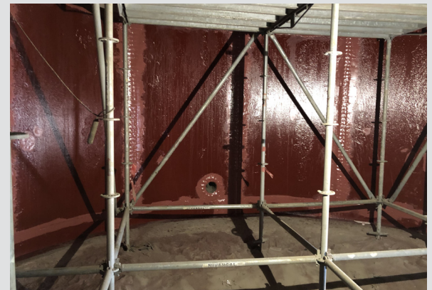
Figure 2 HP-300 Epoxy was installed at 15 - 20 mils and FRP Repair Putty covers the Rivets
