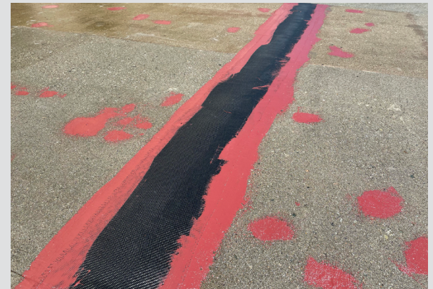
Figure 2 Crack Repaired with Epoxy Elastomer and Carbon Fiber Composite
