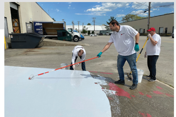
Figure 3 Application of the HP 300 UV Topcoat
