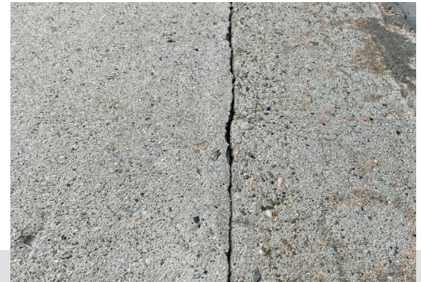
Figure 1 Existing Crack In The Concrete After Power Washing
