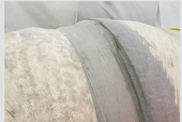
Figure 2 Joint After Leak was Repaired with GF-130 MCU
