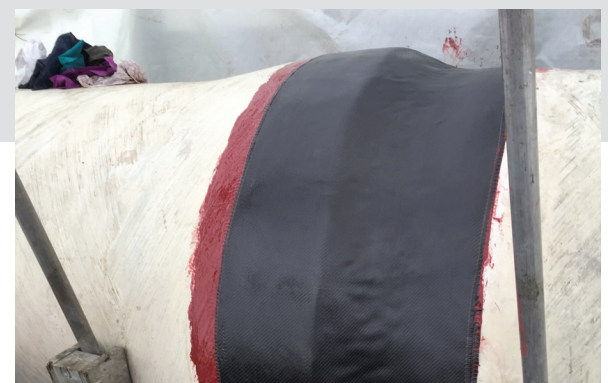
Figure 3 Permanent Repair with High-Strength Carbon Fiber
