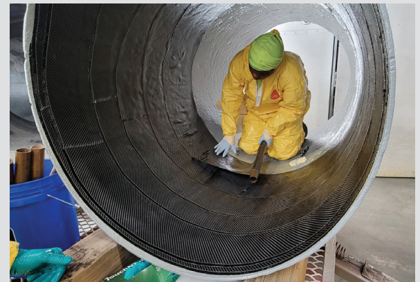
Figure 2 Installation of Carbon Fiber Composite Internal Wrap
