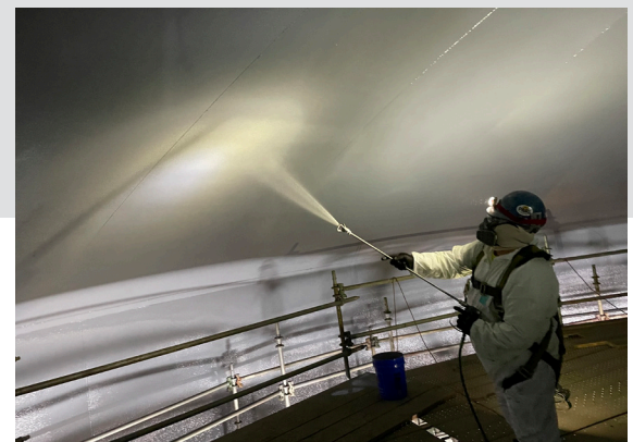
Figure 3 Application of HP 300 GF, an Immersion-Grade Coating System
