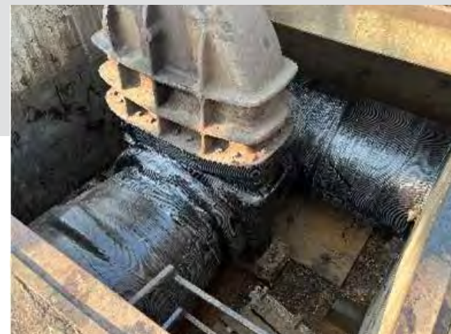
Figure 3 Permanent pipe repair using carbon fiber composites
