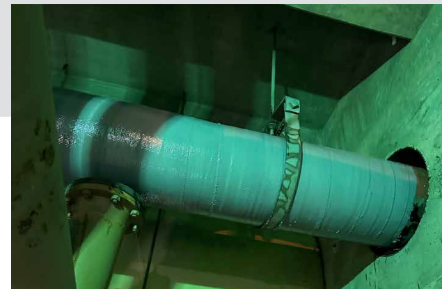
Figure 3 The composite repair system successfully stopped the leaks and reinforced the pipe
