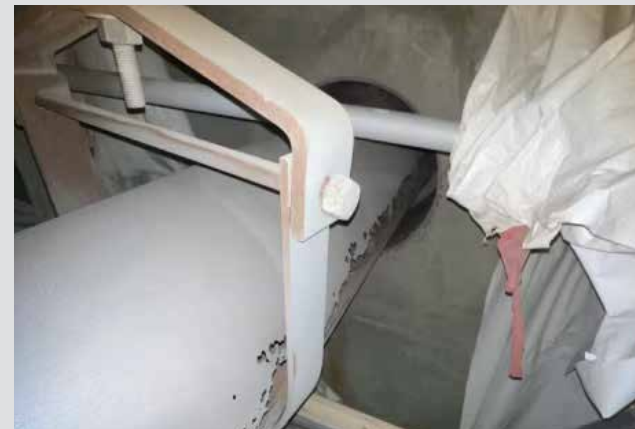
Figure 2 Carbon fiber patches addressed through-wall failures
