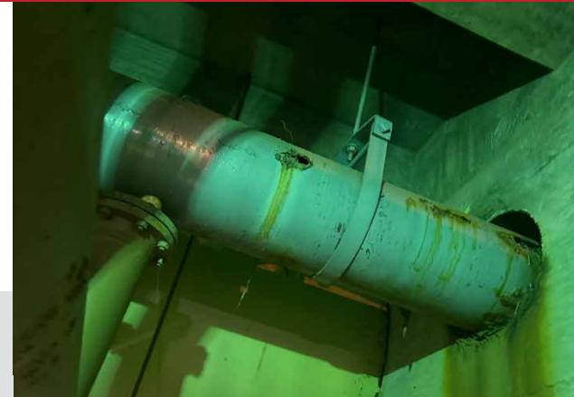
Figure 1 External pipe supports and surrounding concrete walls posed challenges to this pipe repair
